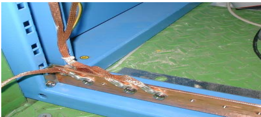
Left and right sides of the rack grounding point
