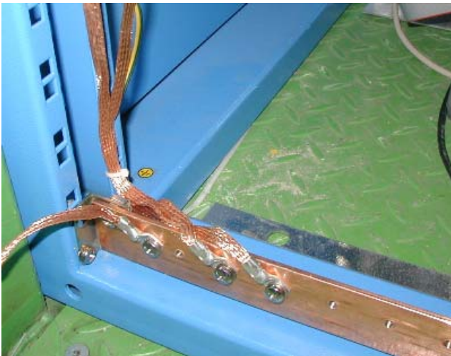
Left and right sides of the rack grounding point
